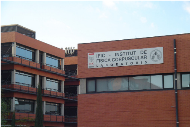
IFIC research buildings at the Science Park UVEG
